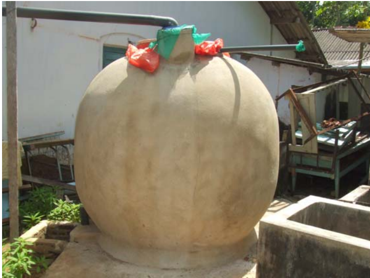
Domestic RWH Water Tank
